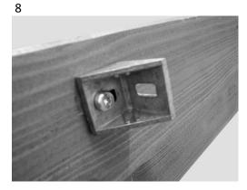
Picture of a ready installed support wire bracket. Align the support wire bracket with the direction of the cord/wire
