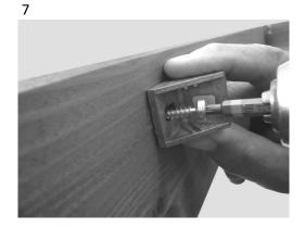
Screw the support wire bracket onto the roofing structure. After the tip of the screw has pierced the aluminium, the thread will grab. **!ATTENTION!**Especially when using thin aluminium do not tighten too heavily
