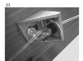
Picture of a ready tied knot of the poly cord. It is absolutely essential that the knot is tightened to a 1,5-2cm knot. The plastic grommet has to be inserted through the washer
